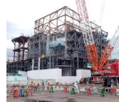
Installing a large cover for Unit 1
