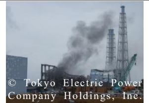
Unit 3 immediately after the hydrogen explosion
