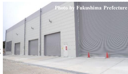
External view of the volume reduction facility
