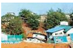
家屋被害：福島市 Housing Damage: Fukushima City
