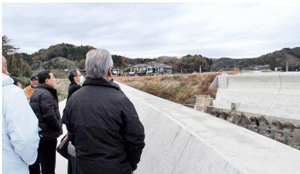
いわき市久之浜末続地区視察 震災後完成した防波堤 Visit to Suetsugi in Hisanohama, Iwaki City Pier Constructed after the Great East Japan Earthquake
