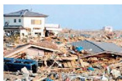
津波被害：浪江町 Damage caused by Tsunami: Namie Town
